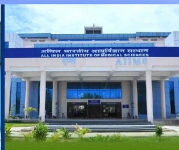
AIIMS Hospital Bibinagar
